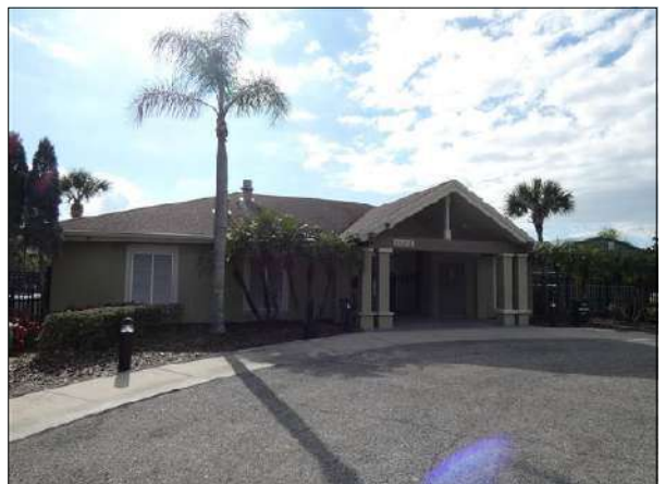
Clubhouse Front View
